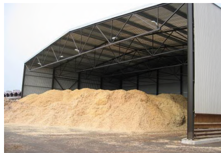
Figure 5.12. Fuel storage – interim storage, (photo Ü. Kask)
