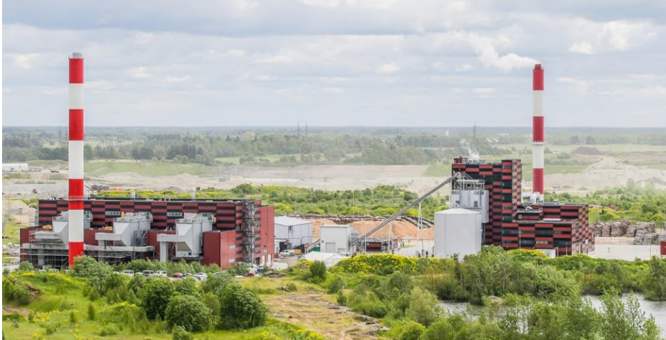
Figure 8.24. OÜ Utilitas Tallinn Power Plant CHP plants in Tallinn, Vao (on the left Vao II, on the right Vao I) [77]
