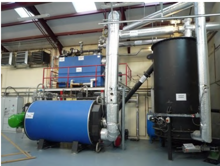
Figure 8.34. Cogeneration station with gasification factor, gas boiler and 35 kW power Stirling engine (Photos Ū. Kask)
