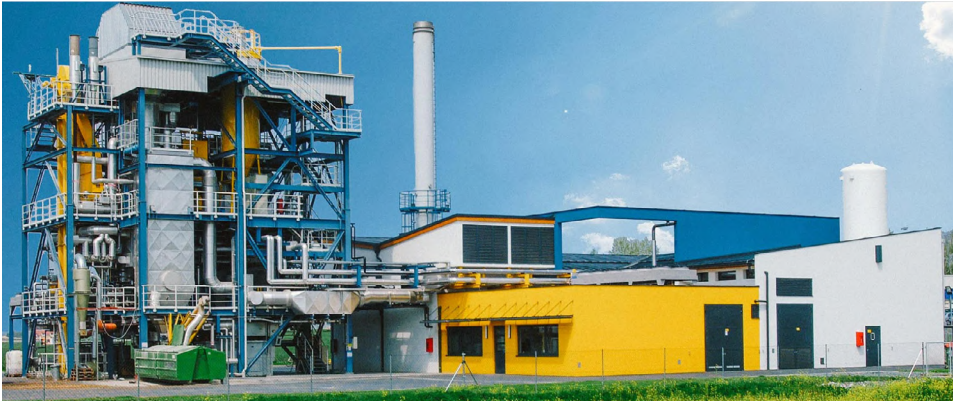
Figure 8.28. CHP plant in Güssing (Austria) with a fluidized bed gas generator and a gas turbine running on local wood industry residues. Electrical capacity 2 \text{ MW}_{\text{el}} and thermal capacity 4.5 \text{ MW}_{\text{th}} [80]
