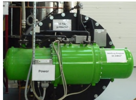
Figure 8.34. Cogeneration station with gasification factor, gas boiler and 35 kW power Stirling engine (Photos Ū. Kask)
