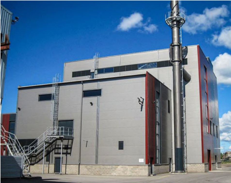
Figure 8.27. AS Kuressaare Soojus Cogeneration plant based on ORC technology and using wood fuel [79]
