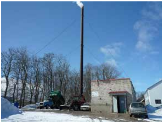
Picture 7. Exterior view of Muhu Liiva boiler house. G
