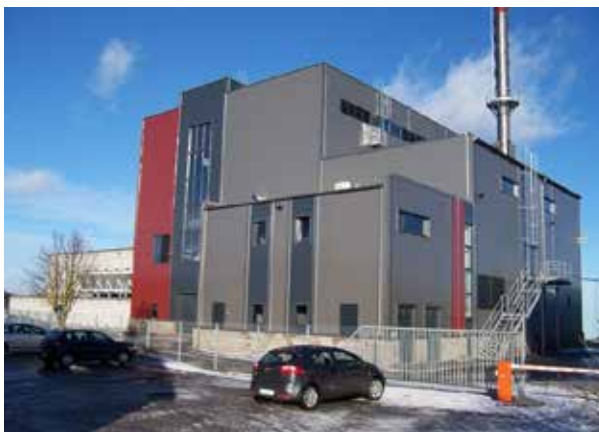
Picture 5. External view of the Kuressaare CHP plant. E
