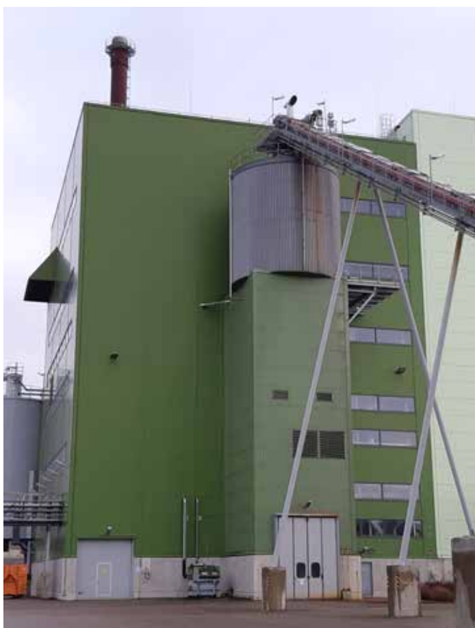
Picture 54. The Finnish listed company Fortum operates the Pärnu CHP plant at the Niidu industrial site. The used fuel is based mainly on wood chip biomass. (Photo: Pasi Poikonen)
